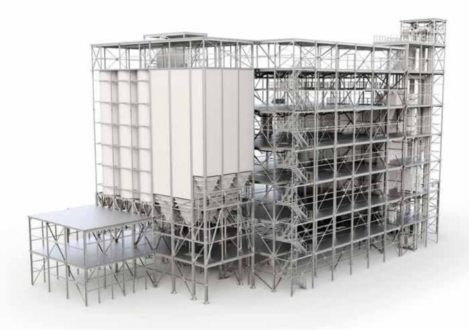
Silos are fundamental components of any storage or processing plant as weighing, dosing, or buffer bins. However, a silo alone cannot ensure seamless plant operation. It requires various accessories and steel structures to ensure functionality and safety, such as supporting or overhead structures and process rooms.
